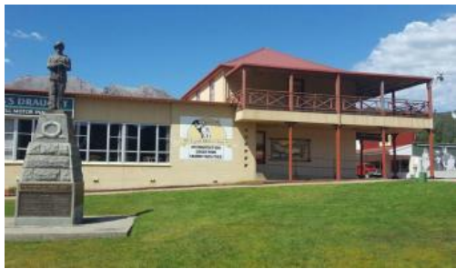
1 Orr Street, Queenstown
